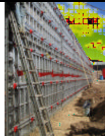
Van Wyk's pouring 18' high wall shop addition with their pump.
