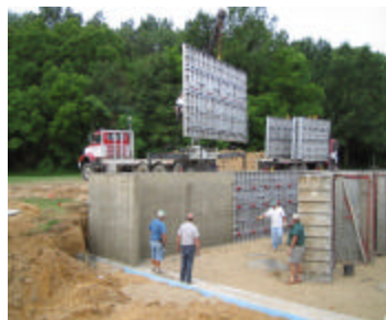
Esker's 9' x 21' long B.E.P being stripped.
