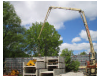
Van Wyk's pouring 18' high wall shop addition with their pump.
