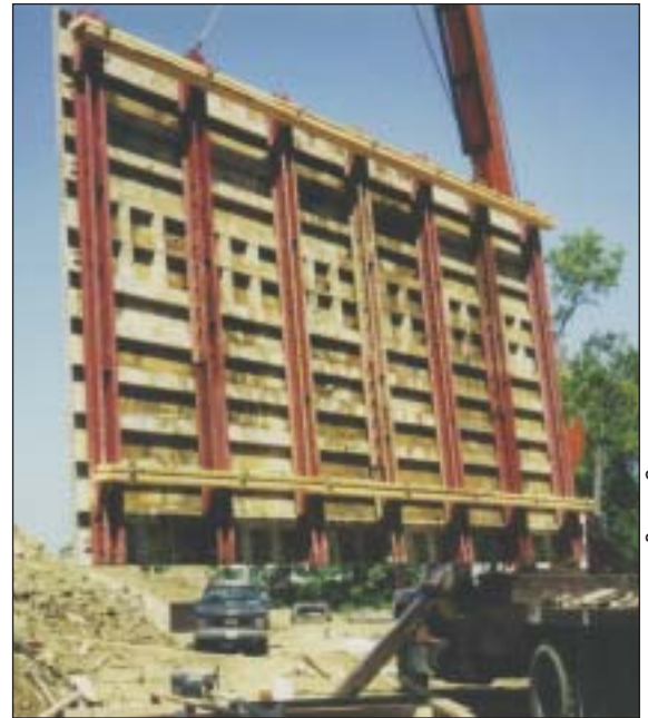
GANGS AWAY (above): For projects with longer wall spans, gangforming can be a cost-effective alternative to handsetting panels, particularly for larger projects or repetitive pours. Here a crane lifts a ganged panel and sets it into place.
